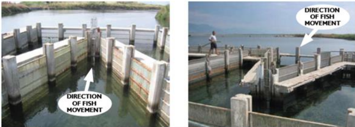
Figure 3. Permanent fish entrapment devices, which catch live fish as they move seawards (Vassova and Erateino Lagoons, Nestos Delta). The arrow shows the direction of fish movement (Source: E.T. Koutrakis).
